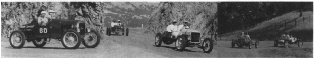
The wheels on Bob Plegge's speedster are quite unusual. They have demountable rims of the Hayes type, and use 30 by 3% tires. The spokes are solid steel and bolt into a regular Ford hub. They are light and quite strong. Bob has been unable to locate any information as to the manufacturer, etc. Reader comment is invited.
