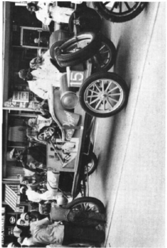
Vic Schmidt's speedster has a mostly stock T engine with a single down-draft carburetor and Bosch ignition.
